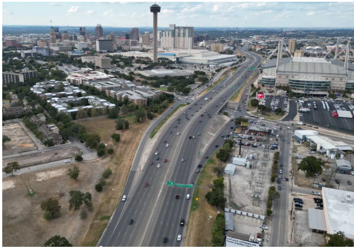
US 281 separating downtown San Antonio from the Near East Side
