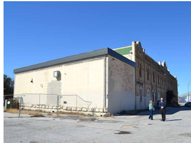
Image: North View of the Rear of the Hugo Building from the South of the Property
