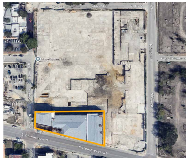
Image: Aerial image of 1617 E Commerce St with Property lines
