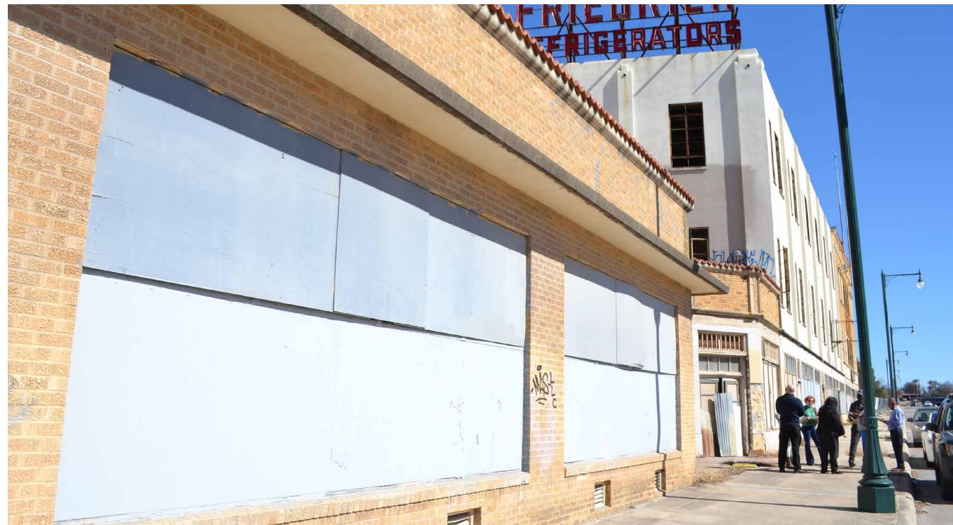
1617 E Commerce The Friedrich Air Conditioning Complex
